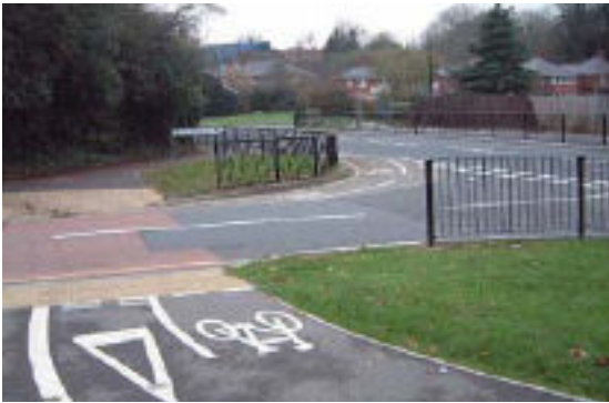
An example of a 'bend-out'. Note the use of coloured surfacing to highlight the crossing, although somewhat excessive use of guard-rails.
