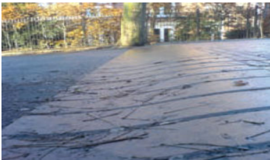
The gentler gradient of a preformed sinusoidal profile ramp.
