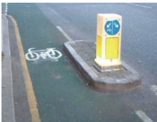
Example of cycle by-pass at a build-out.
