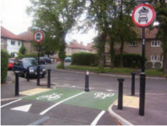
A cyclist exemption from a road closure, using a road hump.
