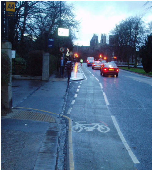
Cycle lane passing side road (diag.1057 is wrongly positioned and should be centrally positioned to the mouth of this minor side road).
